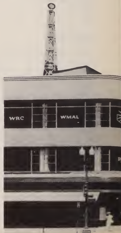
The home of NBC and RCA in Washington, D.C., is the new Trans-Lux Building at 1200 Pennsylvania Avenue.
