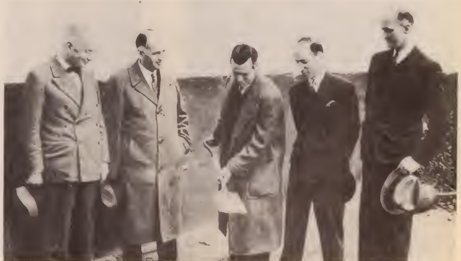
Breaking ground for the new KYW building to be erected at 1619 Walnut St., Philadelphia. Left to Right—William Wark, head of Wark Construction Company; E. H. Gager, KYW plant manager for Westinghouse; Leslie Joy, KYW station manager; Walter N. Gay, representing Hymann & Bros., realtors, and George W. Pepper Jr., architect.
