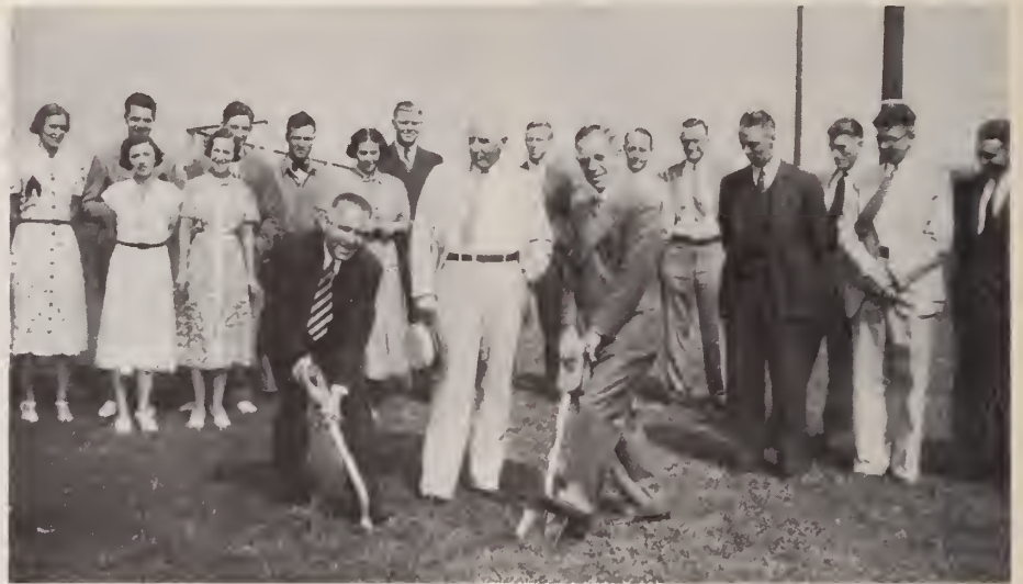
Breaking ground for the new building for WGY Schenectady. Staff members of WGY look on as Kolin Hager, station manager (left) and Chester Lang (right), manager of the G. E. publicity department, break ground for the new NBC studios in Schenectady. In the center, wearing a white suit, is E. E. Talmadge, head of the General Electric Realty Corp.
