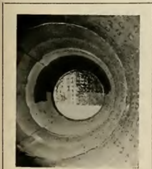
Rubber-Lined Tank Cars for Acid Shipments
