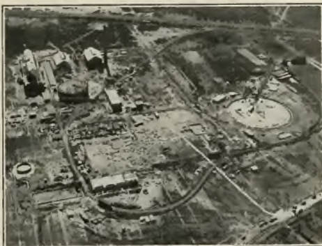
Aeroplane view of the new Mineral Springs Road Plant of the Iroquois Gas Corporation.
