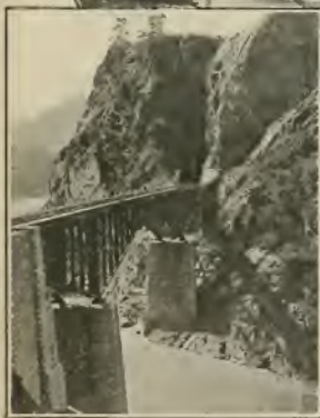
Bridge Construction in the United States Amounted to $133,556,000 Last Year.
