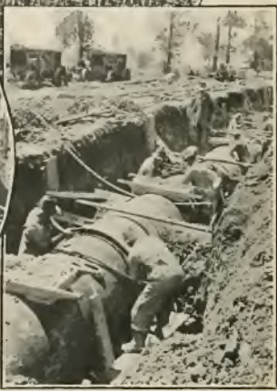
Using Pneumatic Caulking Equipment in Laying Big Water Main.
