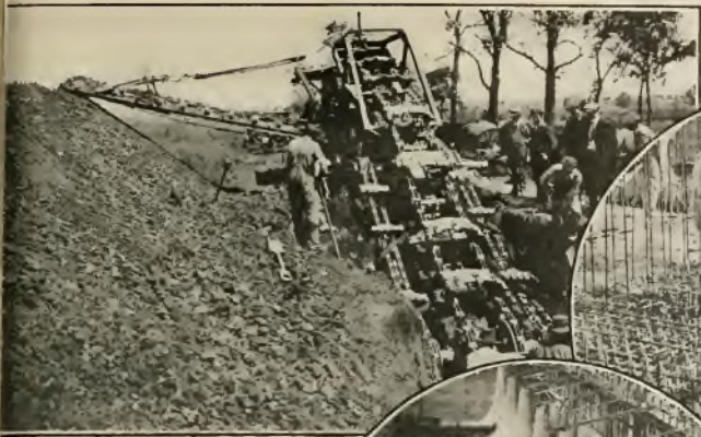
Up-to-Date Trenching Machinery Does the Heavy Work at High Speed.
