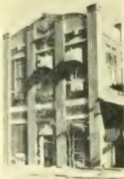
Here is the new office of The Chicago Tribune in Tokyo, Japan. The entire second floor will be used by The Tribune. Roger Matheson, Tribune correspondent in Japan, will make this his headquarters.
