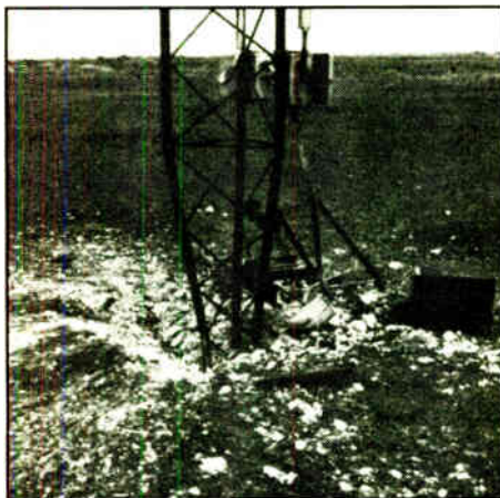
This VOA antenna was driven into the ground from the force of a terrorist bombing, but was not destroyed.
