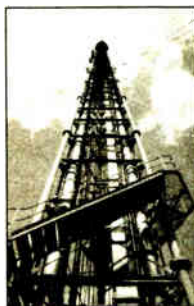
Coaxial Transmission Line
