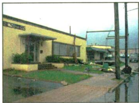
Storm Damage at the Sine Systems Plant in Nashville. See page 3.
