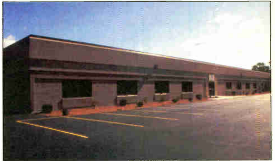
New Intraplex Facility in Littleton, Mass.
