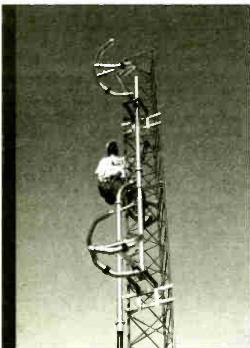
ERI, SHFX series FM Antenna and \lambda Mounting System
