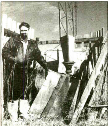
The author is shown at the base of tower No. 6.
