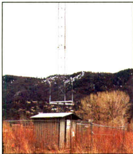
The KIUP (AM) transmitter 'trailer' building is in scenic Durango, Colo.
