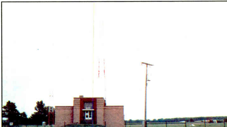
Directional antennas require multiple towers, which are complemented by the radials just below the surface.
