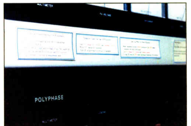
Figure 3: Label transmitter operational procedures to guard against fines and early morning calls.
