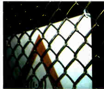
Figure 3: Hang RFR signs inside the fence, but don't use white ties!
