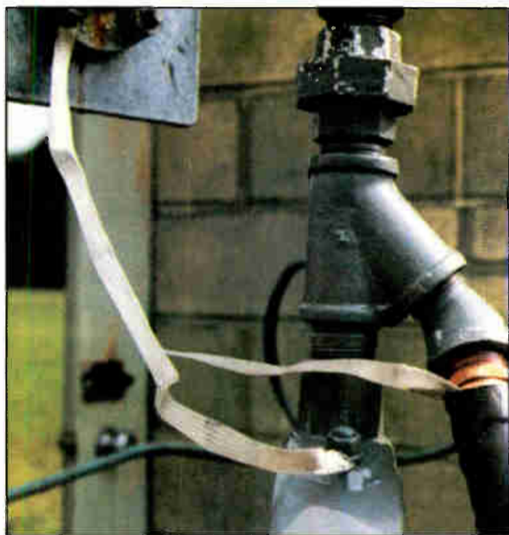
Fig. 1: Using Austin Ring Transformers? Braided wire straps should be connected to a solid ground point.
