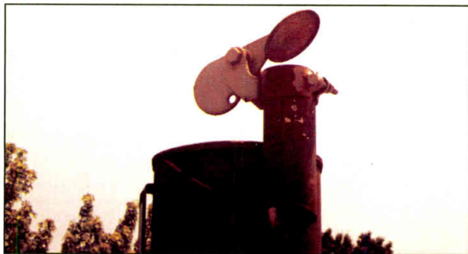
Fig. 1: Make sure the flapper on the generator stack moves freely.
