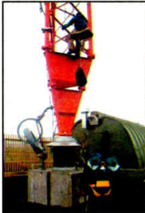
The Base Insulator of the Mast at Eiðar
