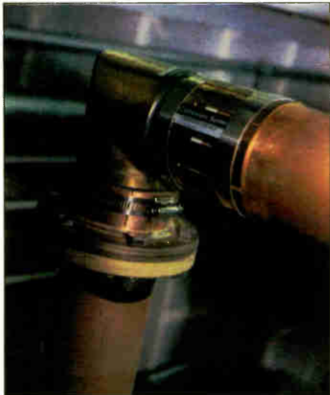
Fig. 3: Clamp-type couplings simplify installation and measurement.
