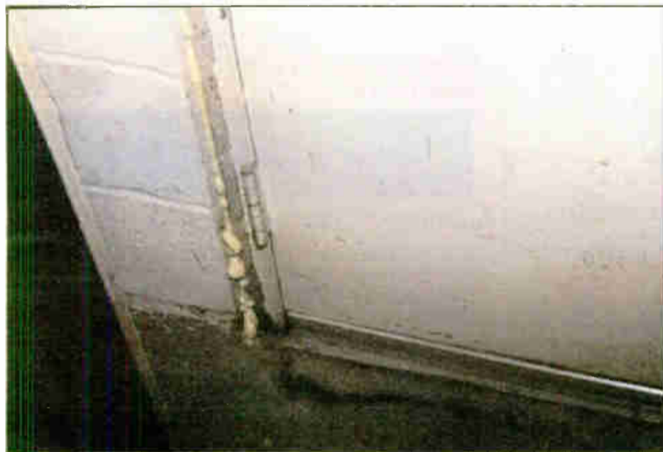
Fig. 1: Spring is a great time to weatherproof your transmitter site ...
