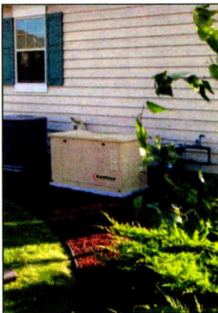
Designed for the North American residential market, the Guardian can be powered by natural gas or Liquefied Petroleum Gas (LPG).
