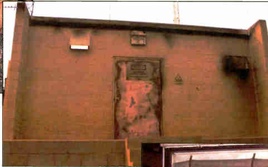
The exterior of the KSGN building.
