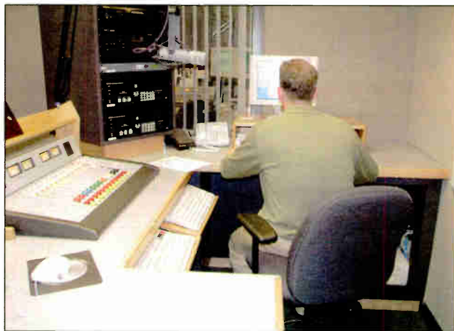
Fig. 2: Cloth-coated vertical blinds like those in the rear of this photo help reduce window sound reflections.
