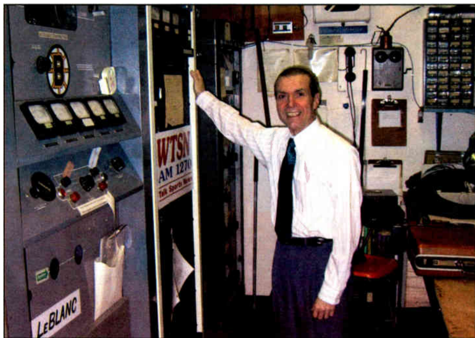
LeBlanc with the station's Harris 5X5 solid state and Gates BC-1J.
