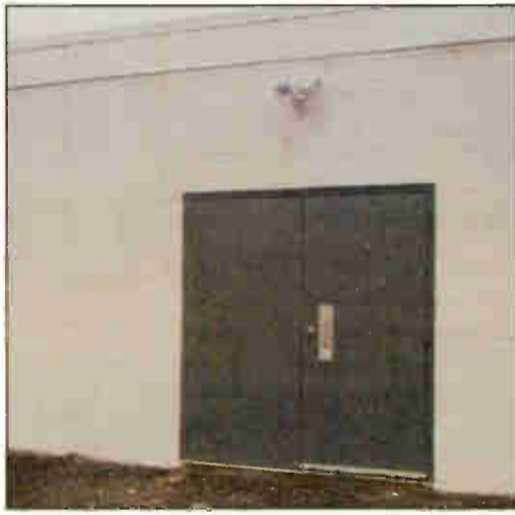
Fig. 2: Double or oversized doors provide easy access for transmitters.
