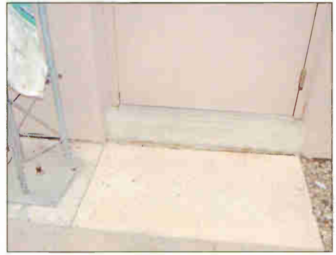
Fig. 3: Measure door and hall entries before the transmitter arrives.
