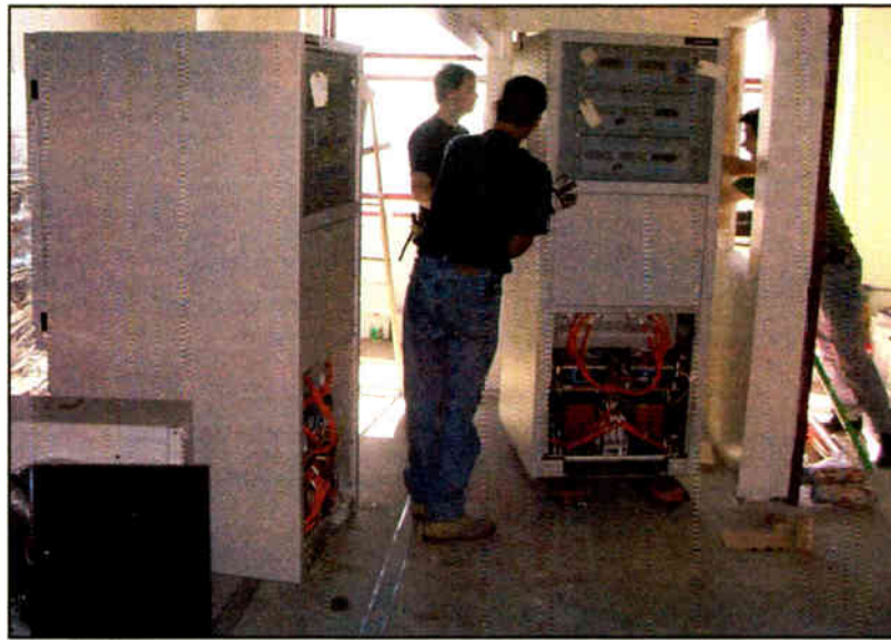
The team wrangles the transmitters into a tight space.
