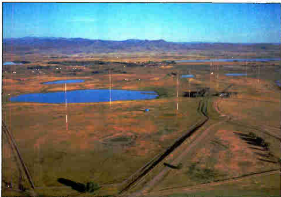
The WWV/WWVB site occupies 390 acres near Ft. Collins. The eight towers of WWVB are prominent, each about 400 feet. Those comprise two capacitance top-hat antenna systems, each with an array of cables suspended from four towers.
