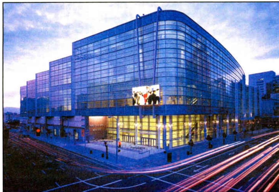
With last summer's completion of Moscone West, San Francisco's Moscone Center covers more than 20 acres on three adjacent blocks.
