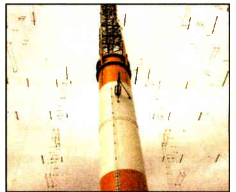
Fig. 6: Wire-Array Upper Mast Detail
