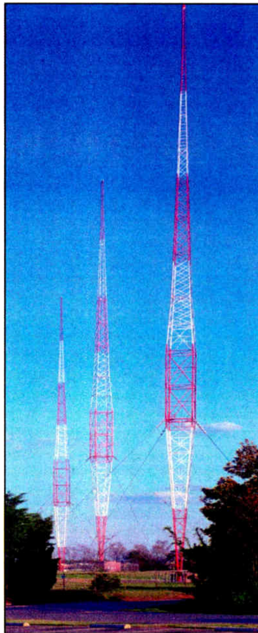
Photo by Scott Fyback, www.fyback.com. Shows: Blount-Knox AM Tower Array at WBT, Charlotte, N.C.
