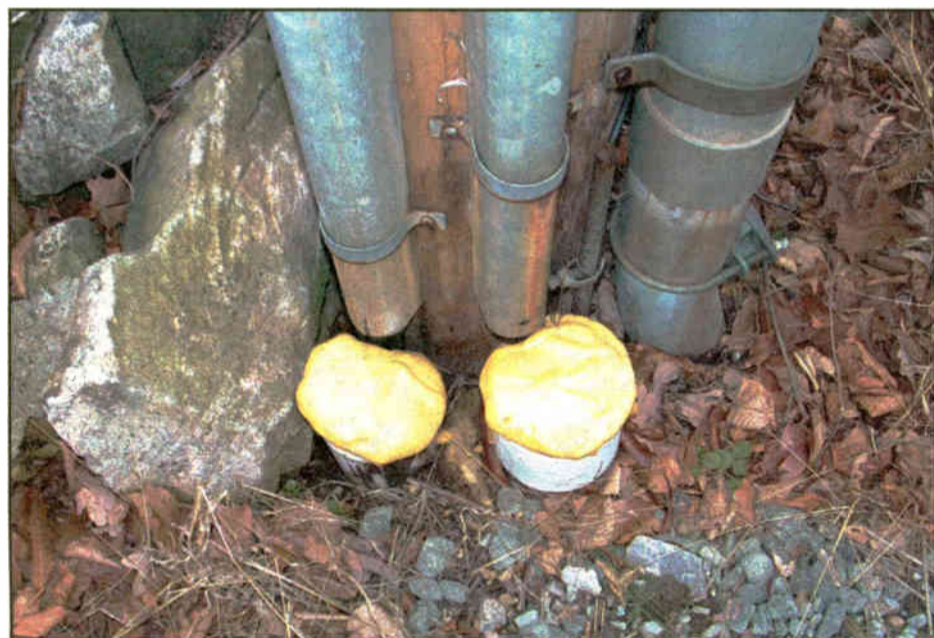
Fig. 2: Use 'dum-dum,' a modeling clay-like compound, for sealing unused conduits.
