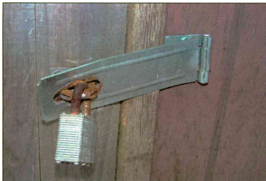
Fig. 3: Install the hasp so it covers mounting screws to deter illegal entry.
