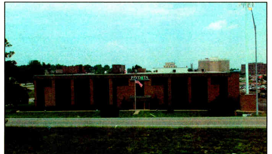
Entercom KC's new home will be in this building in Mission, Kan.
