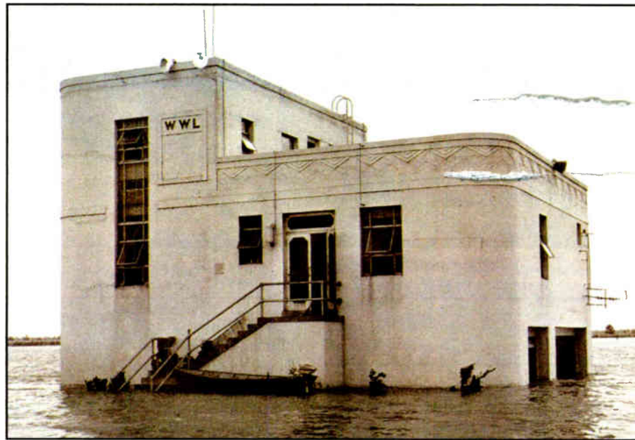
A vintage photo from the WWL Radio archives depicts the aftermath of a 1947 hurricane on the station's former lakefront transmitter site. DOE Joe Pollet says, 'Site access was by boat only, which can be seen tied to the hand rail.' Current images of WWL's elevated, storm-hardened facility also are part of his presentation.
