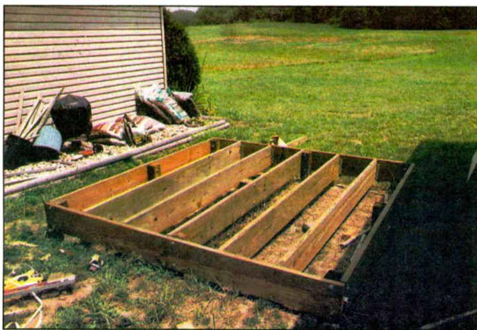
The 2x4 framing for the new transmitter house.
