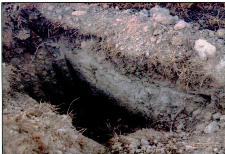
Fig. 1: AM ground radials were damaged due to unauthorized digging.
