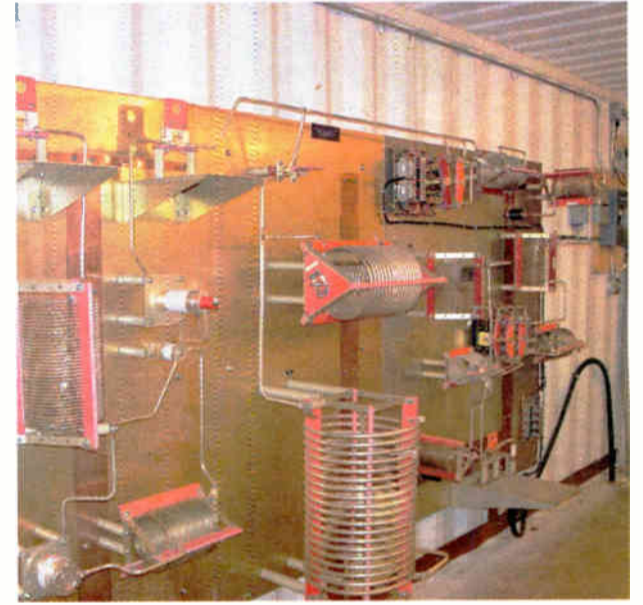
Fig. 3: Securing copper ground strap
