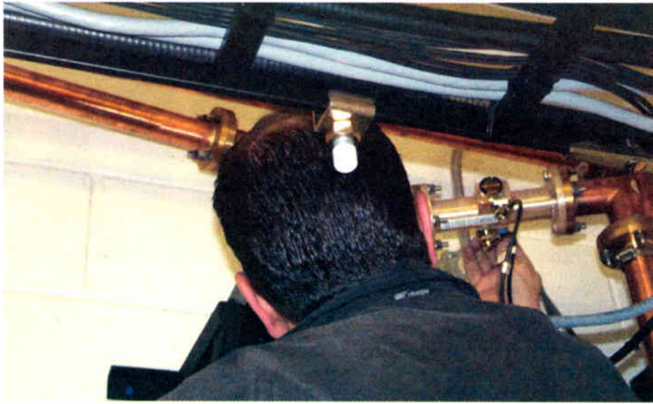
Fig. 4: Slip a plastic nub over that long bolt to save yourself a headache.
