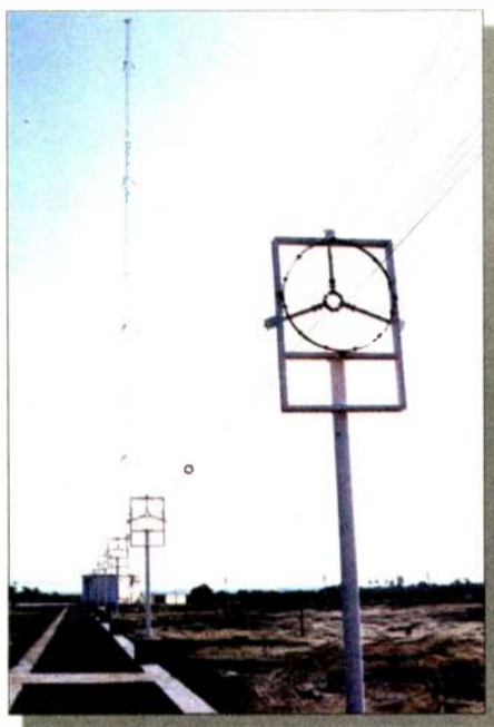
Sri Lanka Open-Wire Transmission Line
