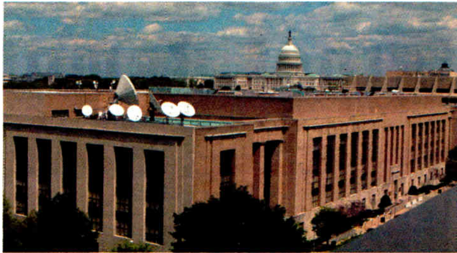
A view of the Cohen Building, VOA headquarters in Washington.
