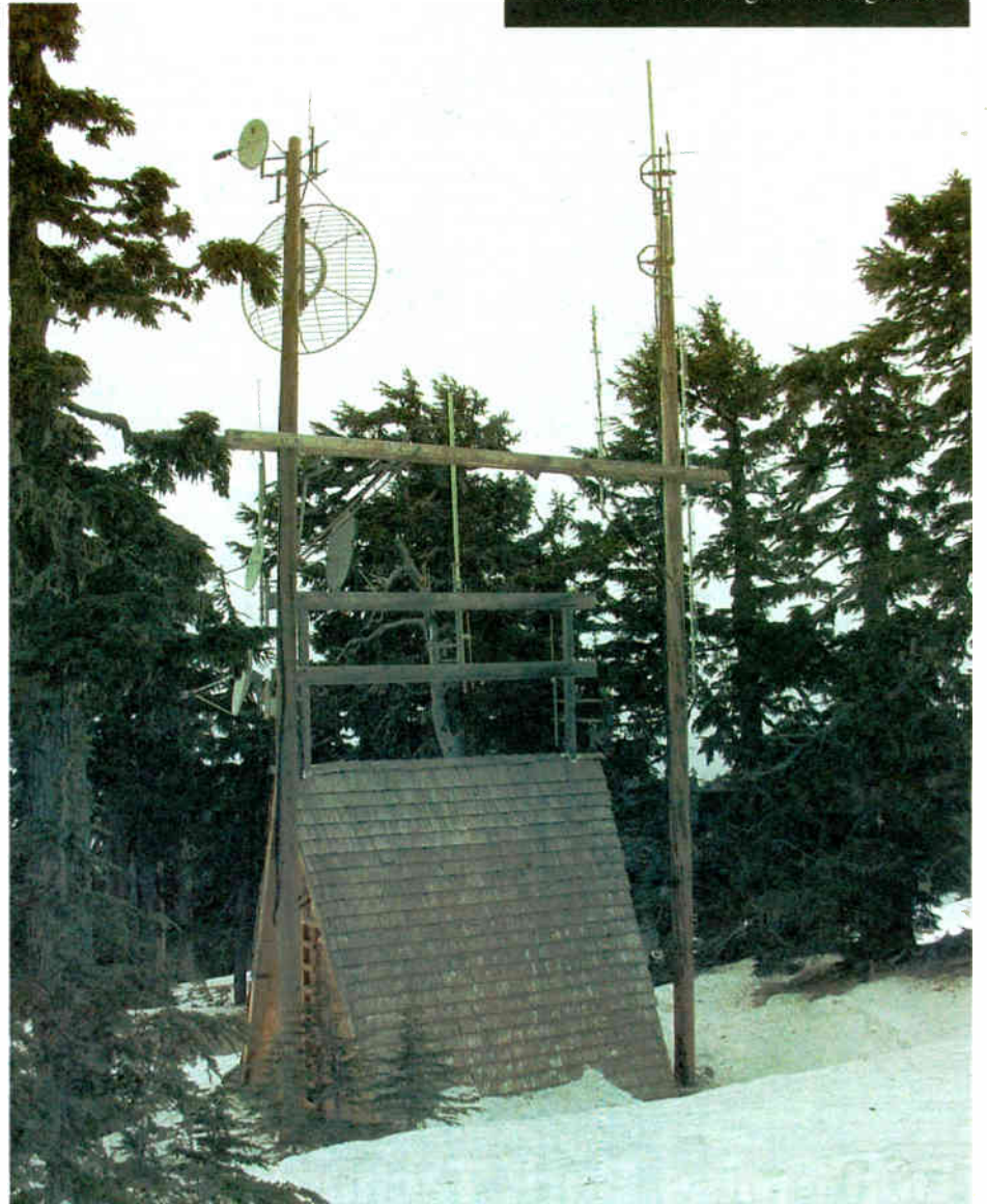
'A-Frame' transmitter building on Mt. Hood, from Jim Dalke's account of the installation of an FM transmitter facility at KPFR with 15 feet of snow on the ground and no landline telephone facility.
