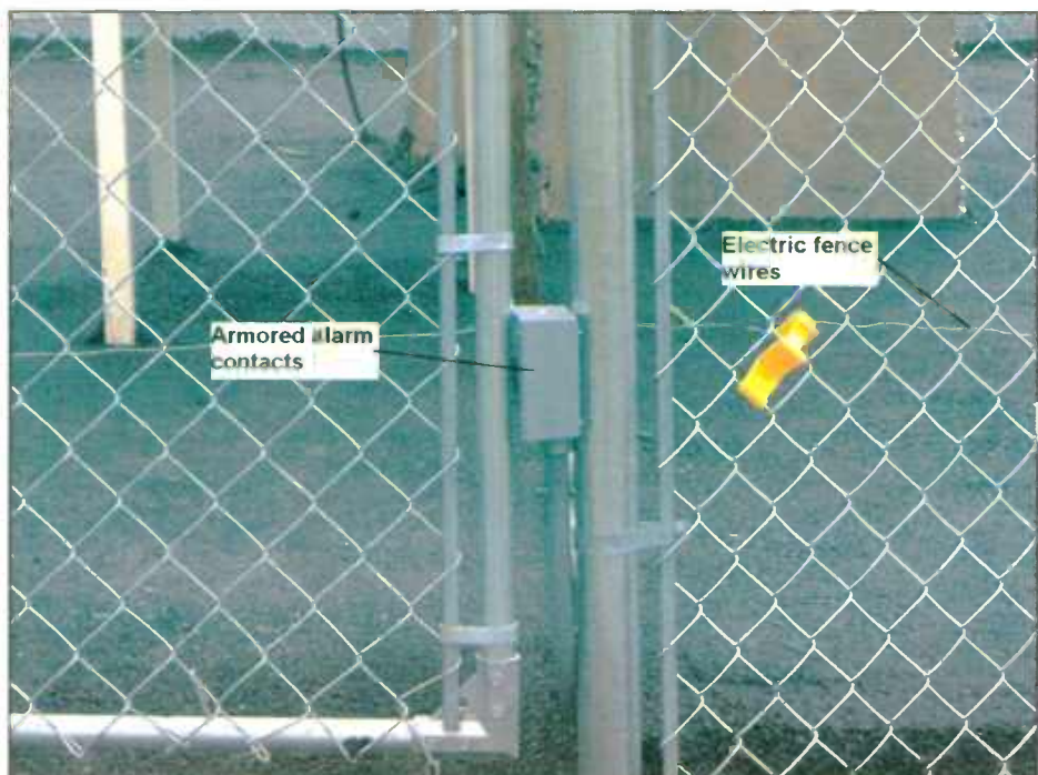
Alarm contacts are enclosed in an armored shell at each tower gate, but even if an intruder smashes the box, the alarm goes off.
