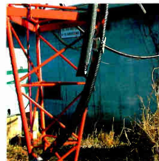
Fig. 2: All that was left was the end of the cut line.
