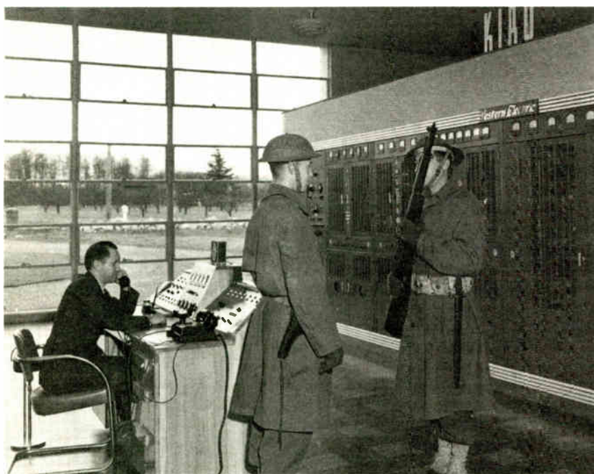
A 50 kW Doherty is visible at KIRO in a 1940s photo. James B. Hatfield Sr. sits at the control console.
