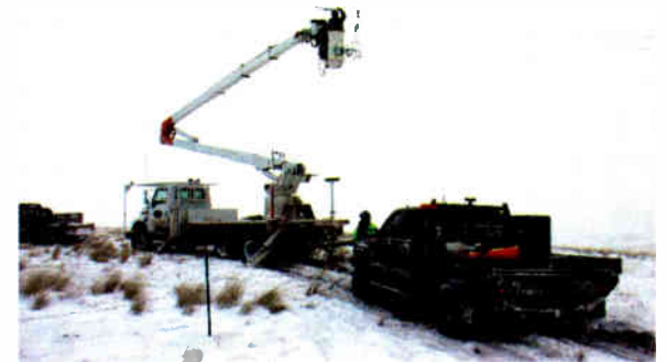
Fig. 2: A lineman makes the connections to connect the generator.
