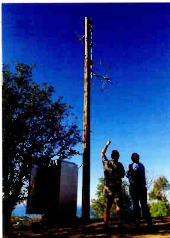
KBUU's scrounged traffic light box. (The station bought it off a loading dock from a California city that had gone bankrupt and had not taken delivery, Laetz says.)
