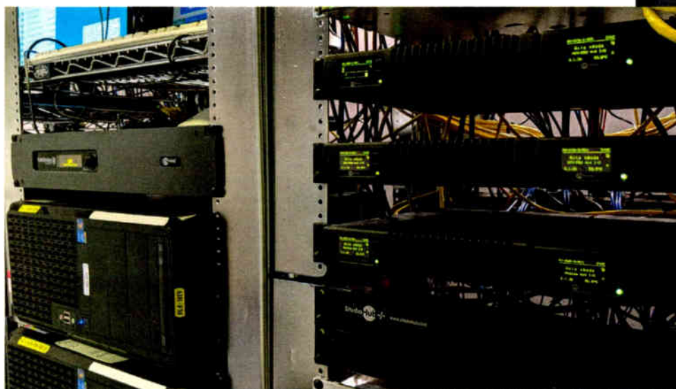
Axia xNodes and the Pathfinder Core Pro in the racks.
