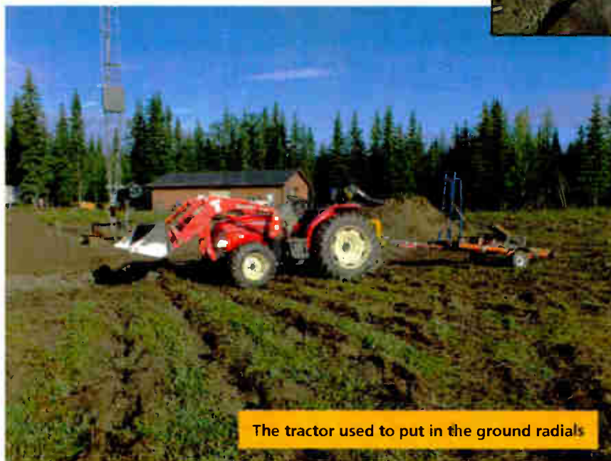
Installing the ground screen
