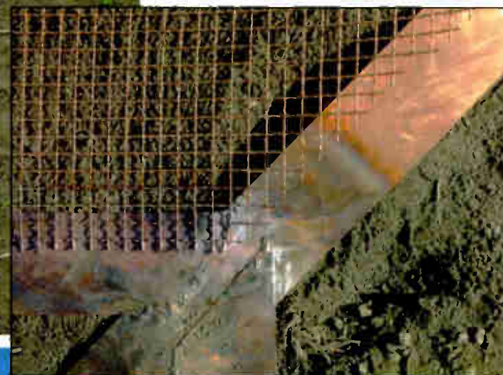
Installing the ground screen
