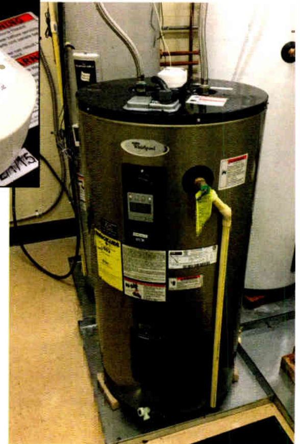
An e-Radio module in action atop a water heater
