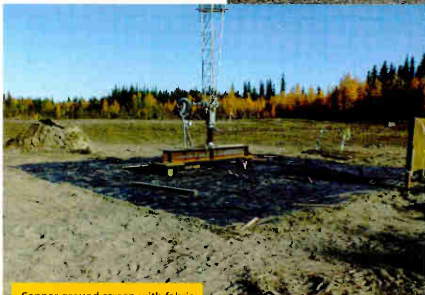
Copper ground screen with fabric
