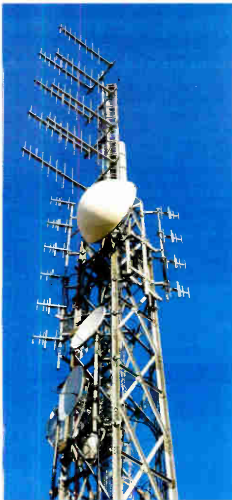
To effectively serve the Piedmont region, a large Kathrein 10-bay, Band III Yagi antenna is top-mounted to the tower. The same tower supports a large, top-mounted Aldena antenna.
