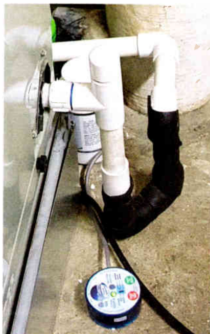
Fig. 1: Pop the cap on the condensate drain and use a flexible bottle brush to clean it out.
