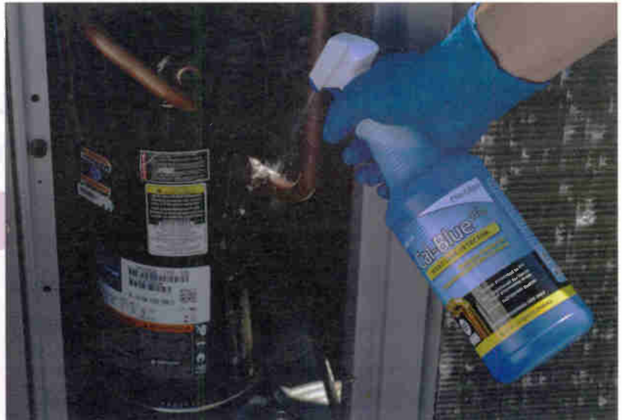
Fig. 3: Cal-Blue Plus stays really gooey for some time after spraying. This makes it easier to spot difficult or very slow leaks.
