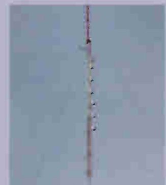
WSEW's new Dielectric antenna is the six-bay system with the white radome covers.
