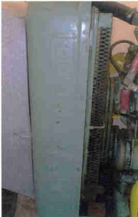
Fig. 2: Inspect radiator hoses like the one at upper right, as well as the belts on the engine pulleys.
