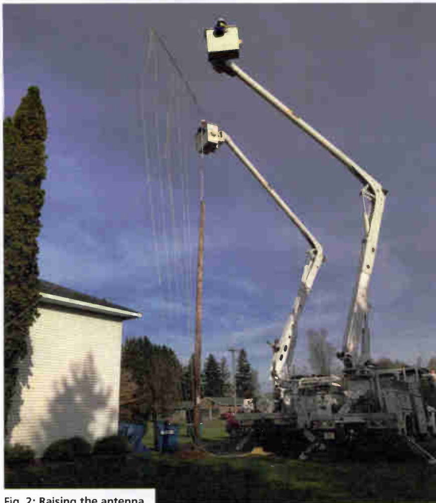
Fig. 2: Raising the antenna.
