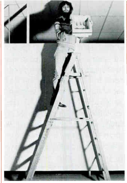
The "SHERMAN SHOCK MACHINE" in Action: Dave Sherman drops the trap samples on concrete floor. Samples were mounted in the open wooden fixture, clamped down to prevent connector damage.
