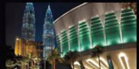
KUALA LUMPUR CONVENTION CENTRE, MALAYSIA 3,000 CAPACITY
