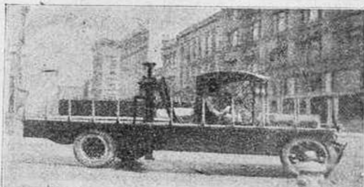
Showing a special truck equipped for setting up tents and driving tent stakes.
