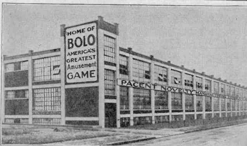
PLANT OF PACENT NOVELTY MANUFACTURING COMPANY, INC., UTICA, N. Y.—Raymond Kay, general manager, says the plant is devoted exclusively to the manufacture of pin games. The Bolo game is made here, from raw wood and metal work to the finished game.
