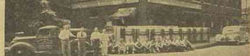
MODERN MUSIC CO., DETROIT, Mills distributor, lines the sidewalk with a shipment of the Mills Throne of Music phonographs. Left to right are Frank McNichols, Don Kelley, Eddie Gramena, Robert Jones and crew.
