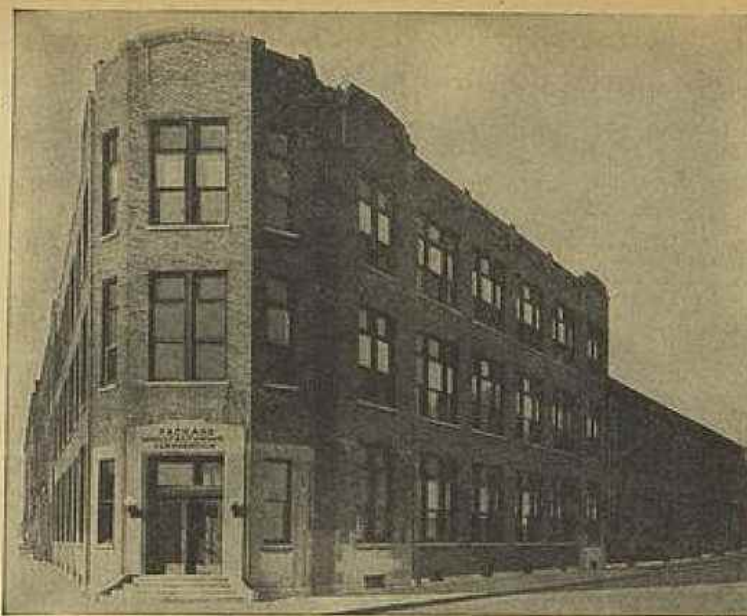
PACKARD MANUFACTURING CORPORATION, headed by Homer E. Capehart, is now installed in this large building in Indianapolis, Ind.
