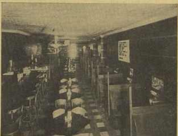
COMPLETE KEENEY INSTALLATION of remote-control equipment in the Holland Mill, Akron, O. The installation was made by the Ed George Novelty Company.
