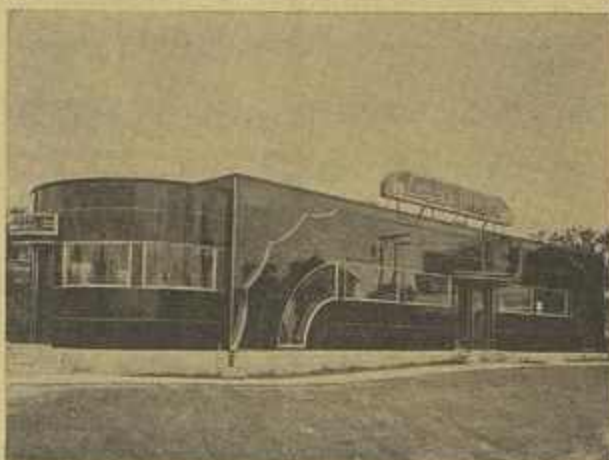
TYPICAL OF THE LOCATIONS which have installed Seeburg Music systems is this diner in Providence, R. I. Seeburg operator I. Wood notes that this diner is one of the most popular spots in the city and attributes much of its favor to the younger set to the remote-control Seeburg installation.
