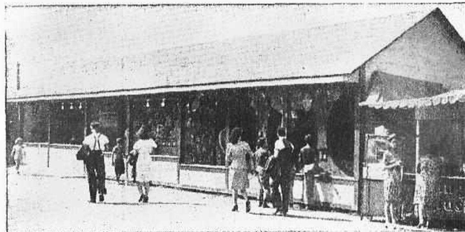
PERMANENT CONCESSION STANDS and paved midways for parks and fairgrounds assuring the acme in sanitation are regarded as a definite "must" by many trade leaders in the post-war era. Pictures above were taken at the Exposition Provincial, Quebec.
